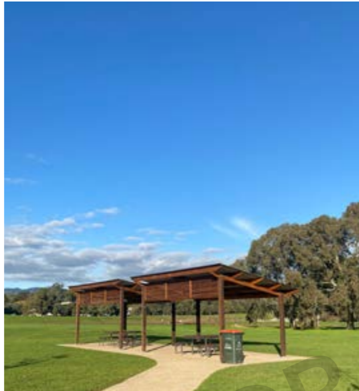
2 New shade structures and picnic settings installed at the Wetland
