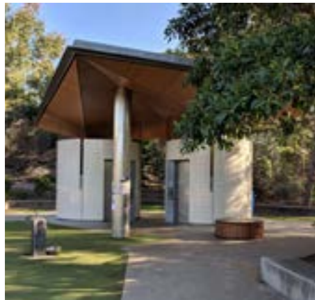
Shade structure with toilet facilities and storage
