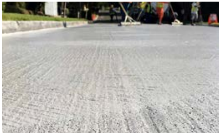
Asphalt cooling spray application
