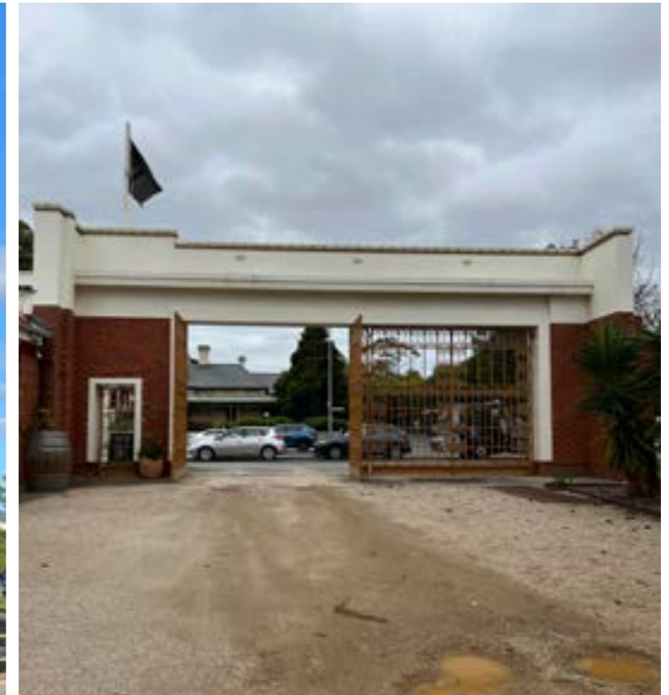
2 Heritage Listed Victoria Park Gates. View through to the very busy Fullarton Road. Gates take visitors to the back of the Grandstand.
