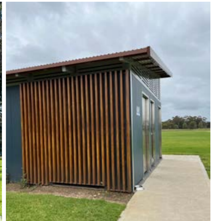
4 Recent, high quality toilet block amenity, installed in the southern half of the park.
